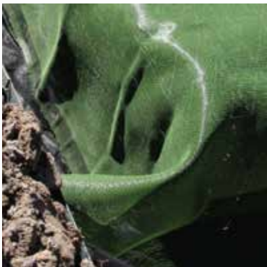
Figure 17: fold corners flat against the tank
